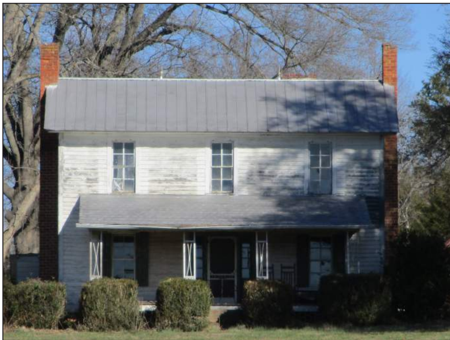
Photograph 2: Facade (south elevation) of David C. Warlick House; looking north. (2017)
