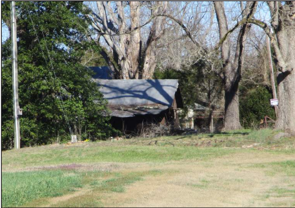
Photograph 6: One-story shed located east of the main dwelling ; looking northwest. (2017)
