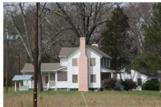
Photograph 12: Edward M. Rozzell House. (2017)
