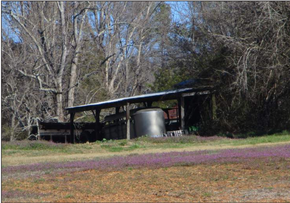
Photograph 10: Shed-roof overhang of the one-story front-gable outbuilding located northeast of the David C. Warlick House; looking northeast. (2017)
